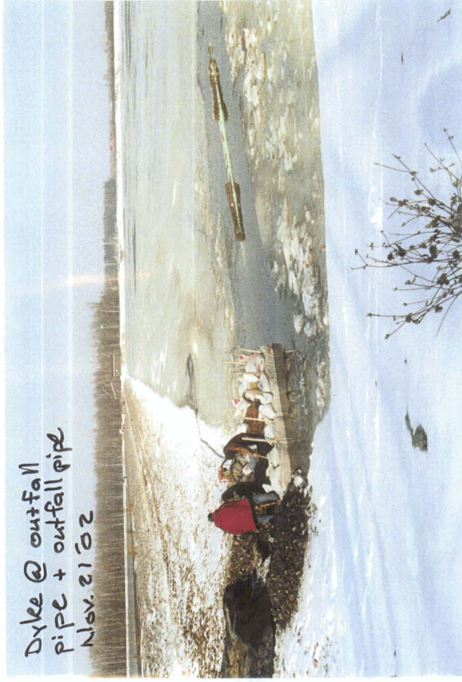
Dismantling of dyke outfall pipe @ proper grade
