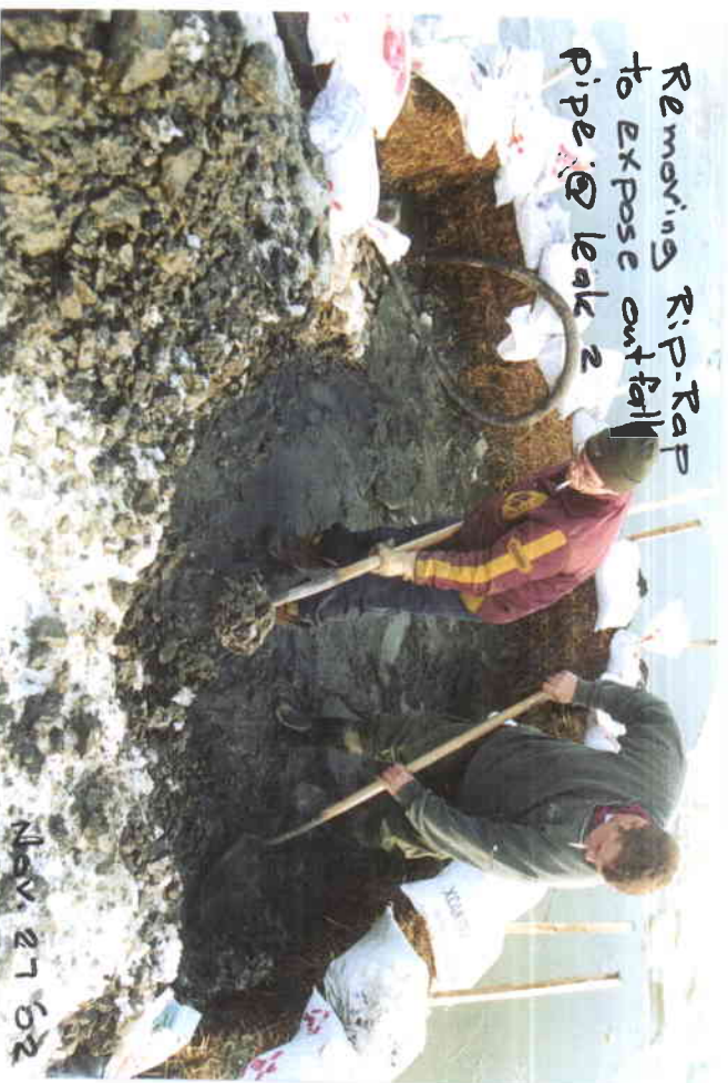
Removing R.P.-RAP @ leak 2
