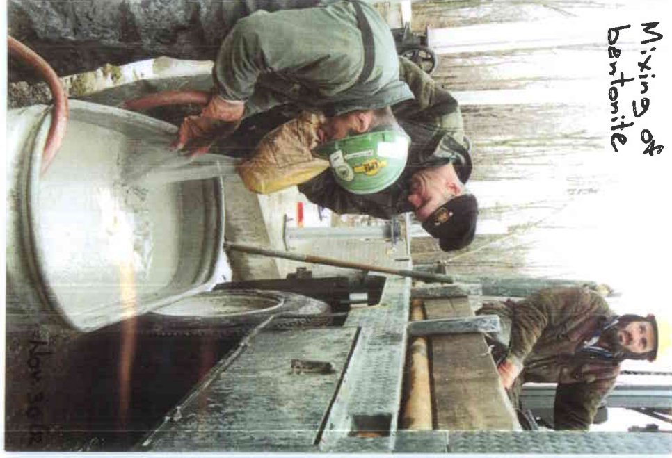
Drill hole 1 for bentonite @ type 2 chamber
